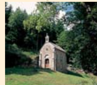
Chapel of Saint-Colomban
